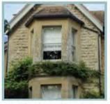
Double storey bay window with glazing set back into the walls to add relief.
